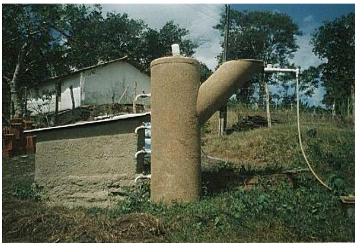
FIGURA 3. Reator UASB
